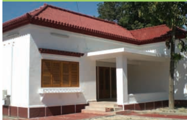
Refurbishment of the residence of MoE, Timor Leste
