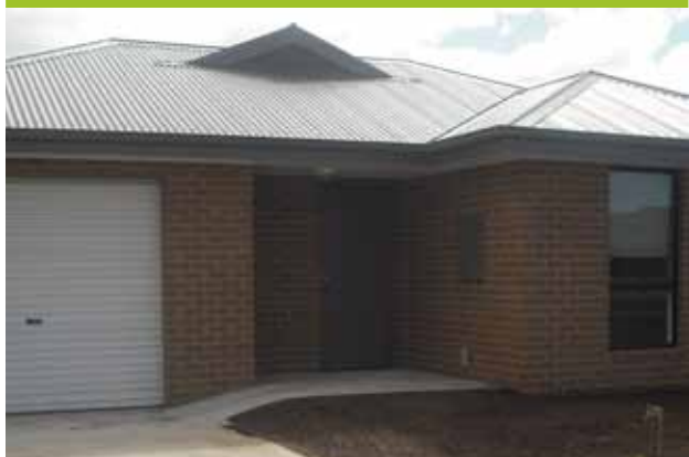
CHL Design and Build property
