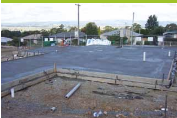
CHL Construction Site
