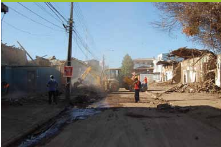
Historic Centre of Curico destroyed due to the Earthquake
