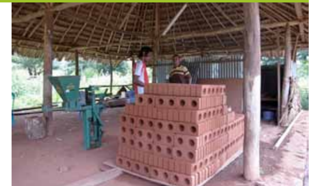
Clay-bricks production unit
