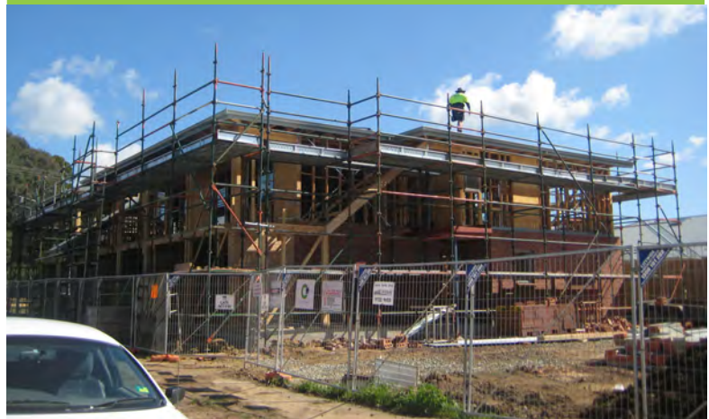
Work well underway at Marine Pde, Hastings, VIC
