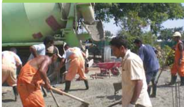
Construction Work underway at a site in Timor Leste
