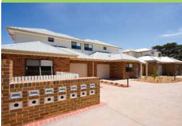
Wentworth Lane Caroline Springs – front view
